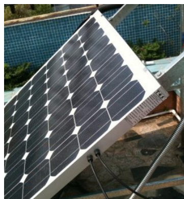
Photos of installation of one PV-T panel for electrical production and daily production of 120liters of hot water at 60 degrees Celsius
