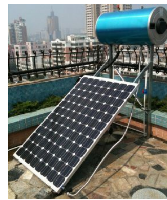
Photos of installation of one PV-T panel for electrical production and daily production of 120liters of hot water at 60 degrees Celsius
